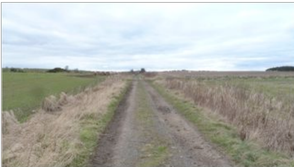
Route section on dismantled railway used as farm track
